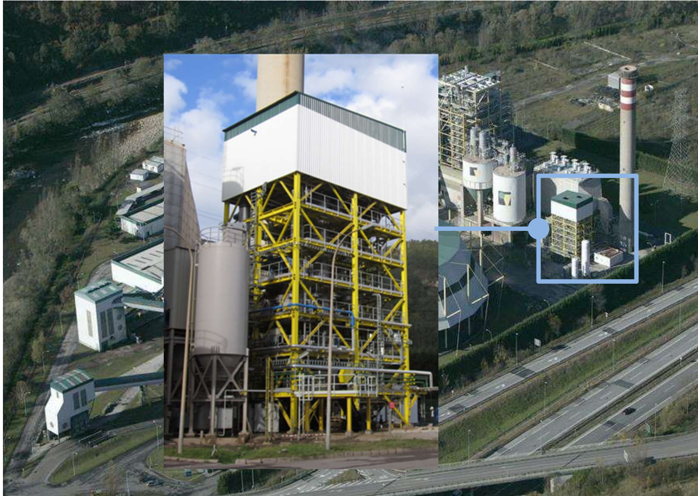
Reactors: 15 m height, 0.7 m i.d.
