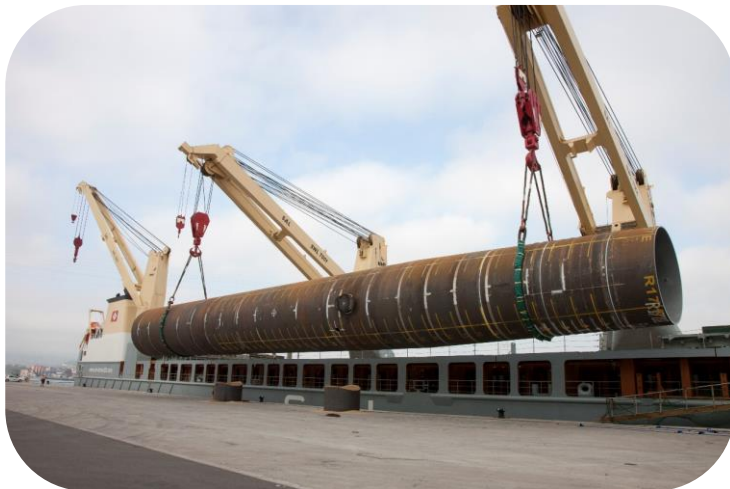
30 MONOPILES OFFSHORE WIND (~24.000 TON)
