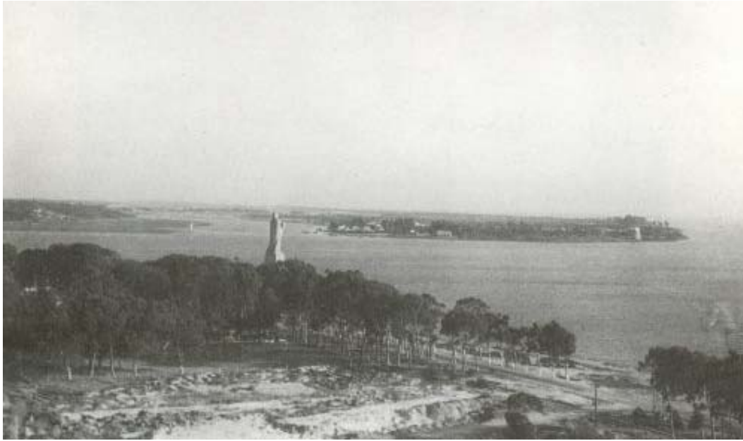
View of "Nuevo Puerto" And Domingo Rubio's Tideland from the Punta del Sebo before the implantation of the industry and the bridge Foto C. P.
