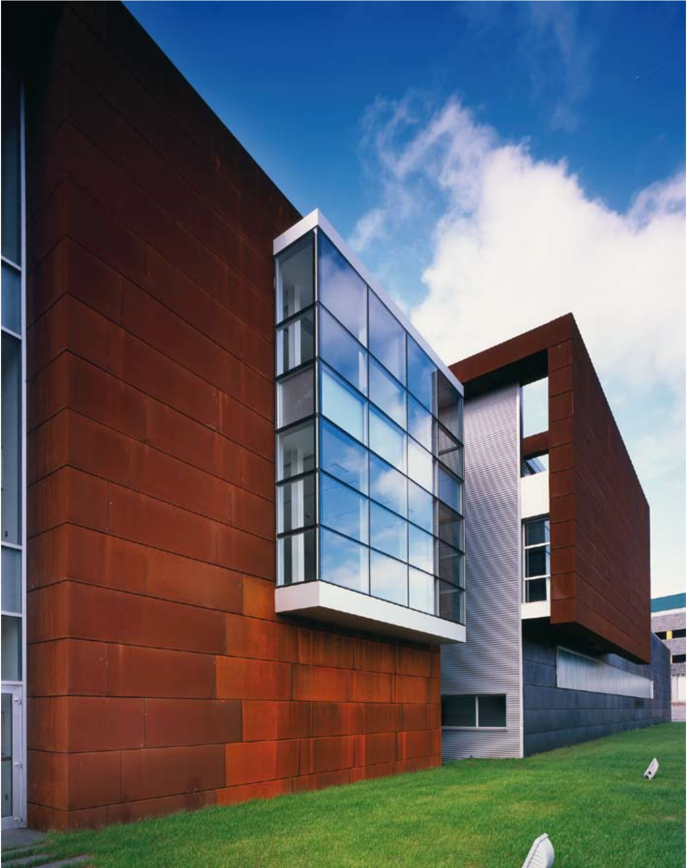
Steel Technology Centre.
